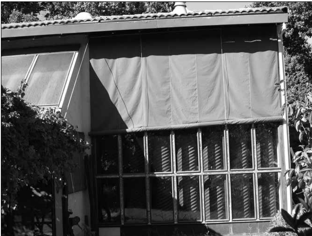
Figure 2.—This passive solar “suncatcher” house has large, metal, fluid-filled pipes that provide thermal mass. To the left of the photograph is a greenhouse-like room behind the grapevines.
