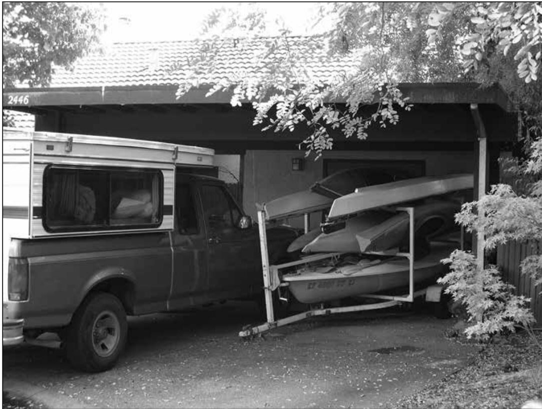
Figure 4.—As part of the effort to de-emphasize the automobile, only forty-nine dwellings have garages and 140 have only carports. Further, twenty-nine residences have only uncovered parking. One result is a more cluttered, in some cases messy, streetscape.
