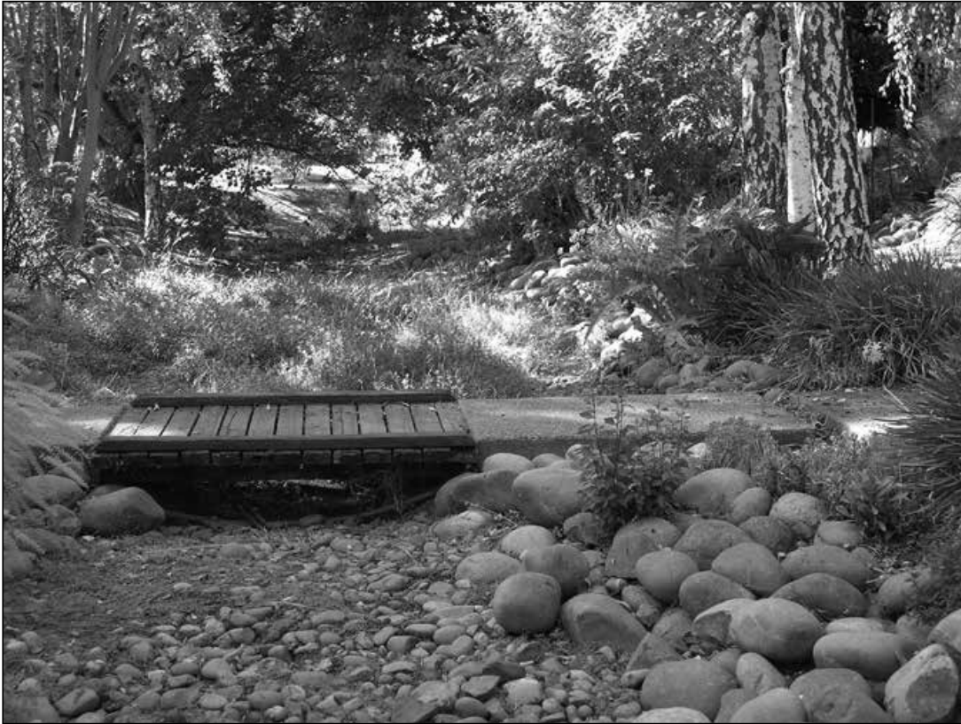
Figure 9.—A small bridge crosses one of many low-lying areas that serve as part of Village Homes’ innovative surface-drainage system. Thirty-five bridges, large and small, are functional and aesthetic landscape features.
